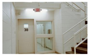
The Quasar Exit Sign & Emergency Combo is the perfect choice when space is at a premium. The combination exit and emergency lighting has a self-diagnostic option available. It is ideal for applications requiring quick installation of both exit sign and emergency light. Each unit has a streamlined design for above-the-door applications and other tight fits. This combo exit & emergency light delivers 25' center-to-center spacing to meet the NFPA 101 Life Safety Code with fewer fixtures.
