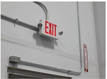
The Exit Sign Combo combines the classic exit sign with a pair of flood lights, in a single fixture. The battery backup provides more than 90 minutes of emergency operation for safe building egress and code compliance. The 5W input wattage recharges the unit within 24 hours of battery backup use. The unit is designed for fast and easy wall mounting to a standard J-box.
